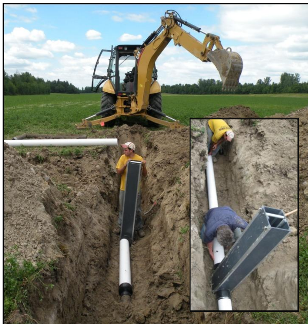
Figure 2: Installation of a water control structure in a field at the Miner Institute.
